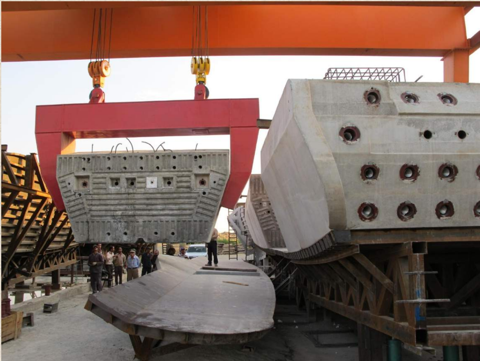
Precast – Pre_stressed Cap Beam
