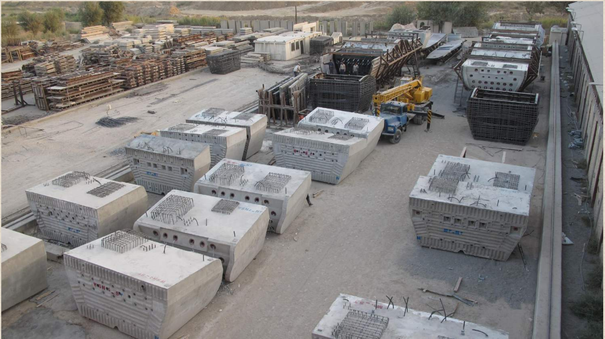
Precast – Pre_stressed Cap Beam Tehran - SADR Elevated Highway (2012)
