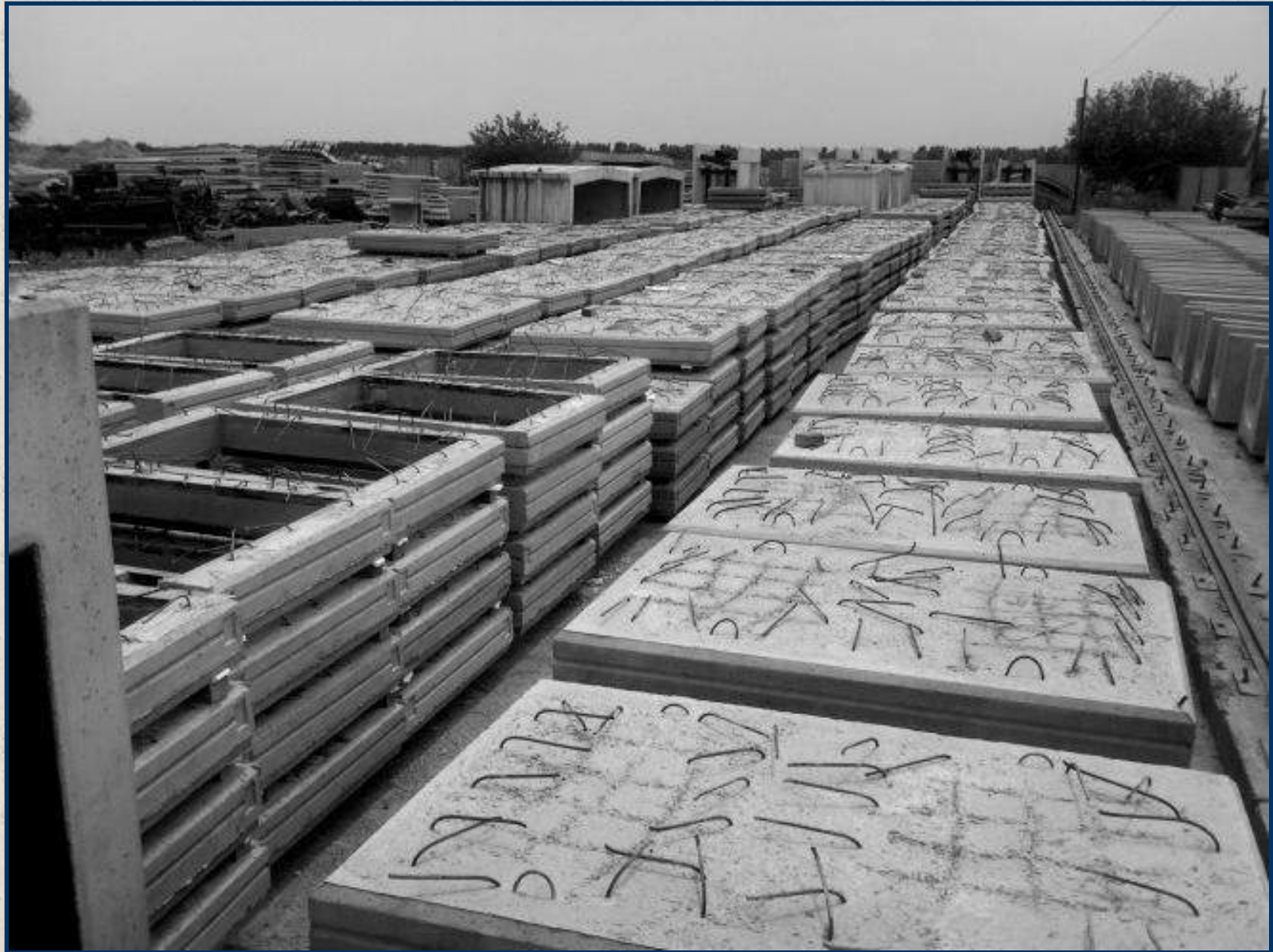
Traffic Tunnel Precast Elements - MKBeton Factory
