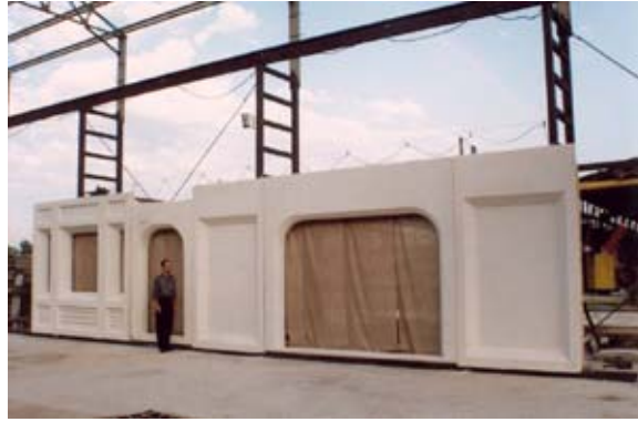
A combination of sand-blast finish of structural facades using white concrete
