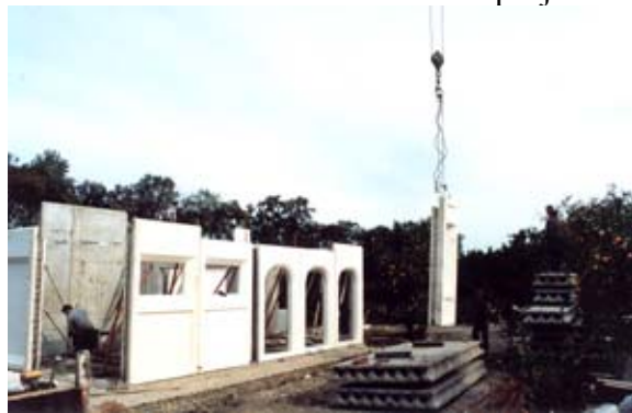
A window panel is being erected by the crane
