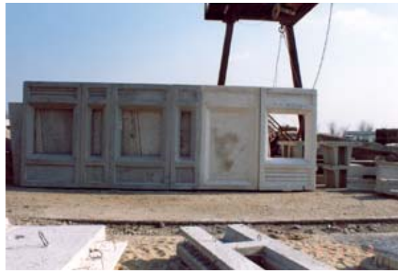
A combination of structural facades erected in the factory
